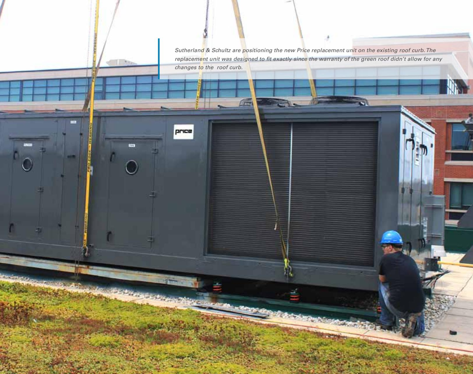
*Sutherland & Schultz are positioning the new Price replacement unit on the existing roof curb. The replacement unit was designed to fit exactly since the warranty of the green roof didn't allow for any changes to the roof curb.*
