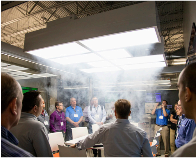
The Price Technical Center features our Ultrasuite® system, an operating room diffuser system with integrated LED lighting
