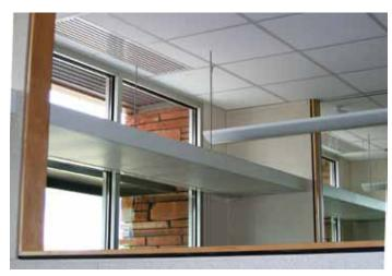
efficient benefits of other radiant panels. Light Shelf Radiant Panels can be installed directly onto window mullions for a seamless look, or combined with other options such as a bullnose profile, to achieve a unique design. The top cover can also include an active radiant top to increase the energy capacity and surface area of the panel. A Price Light Shelf Radiant Panel can be designed to fit your needs and space requirements.
