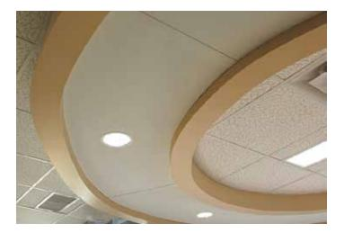
architectural requirements. Cut-outs for lights, sprinklers, grilles and registers can be integrated into panel construction to save ceiling space and improve aesthetics. Other options include panels hidden within structural building supports, smooth faced aluminum or heavy duty steel vandal resistant security panels, or curved panels.
