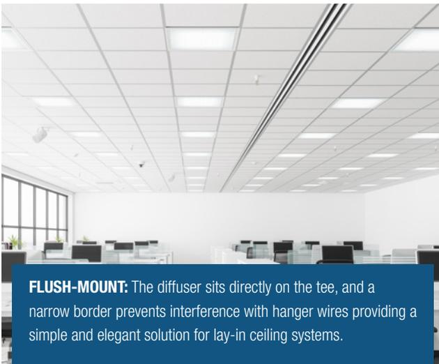
**FLUSH-MOUNT:** The diffuser sits directly on the tee, and a narrow border prevents interference with hanger wires providing a simple and elegant solution for lay-in ceiling systems.
