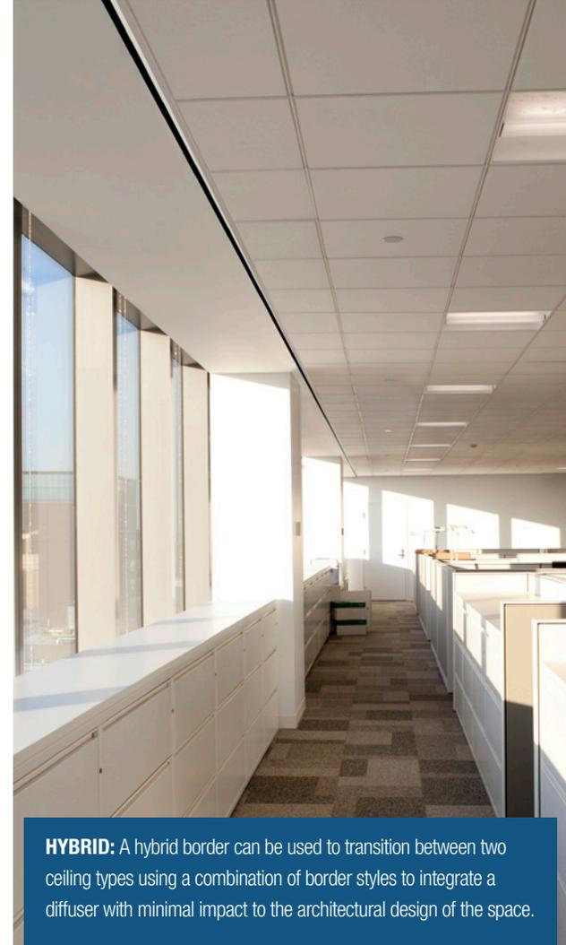
**HYBRID:** A hybrid border can be used to transition between two ceiling types using a combination of border styles to integrate a diffuser with minimal impact to the architectural design of the space.
