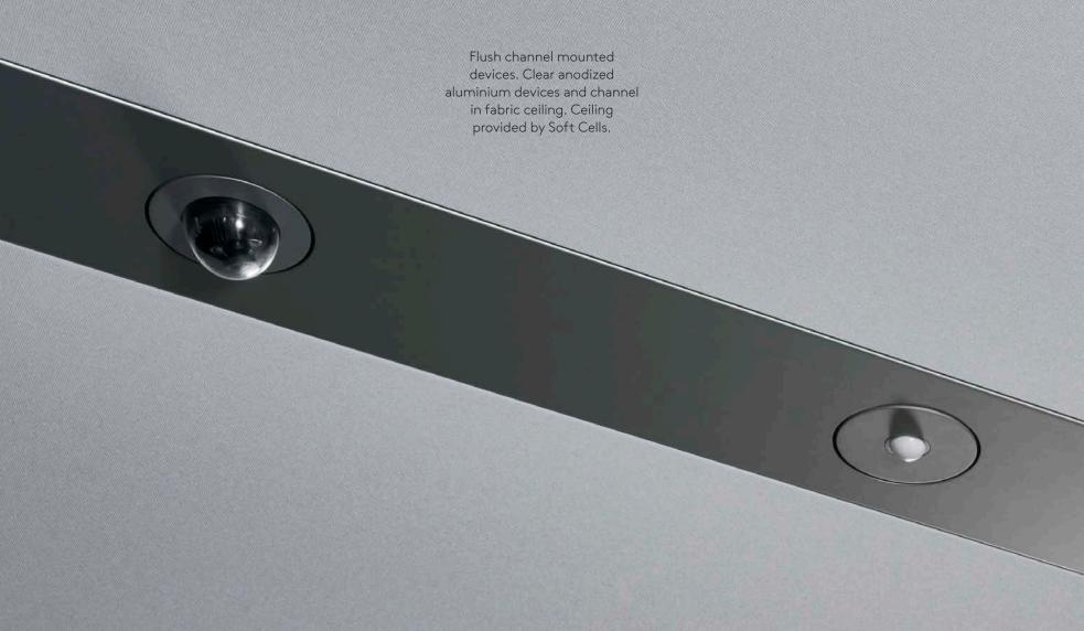
Left to right: Security Camera, BACnet Multisensor, Emergency Light
