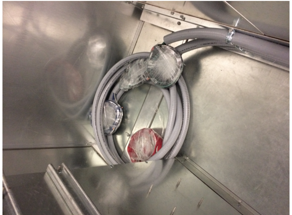
FIGURE 7: HIGH VOLTAGE WIRES SPOOLED ▼
