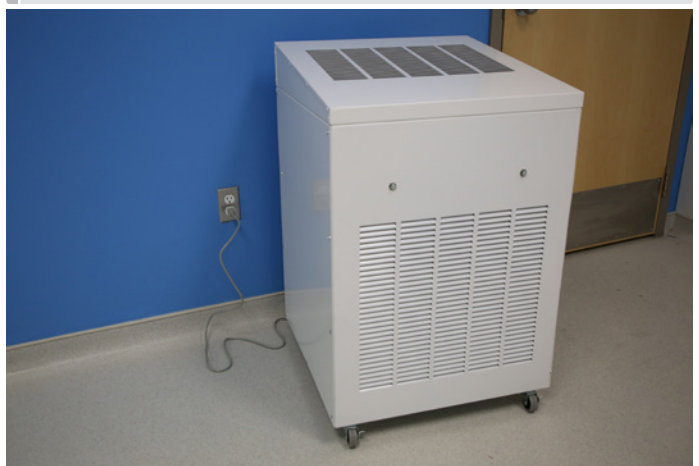
THE RAP, PLUGGED IN AND FACING TOWARDS THE OCCUPIED ZONE ▼
