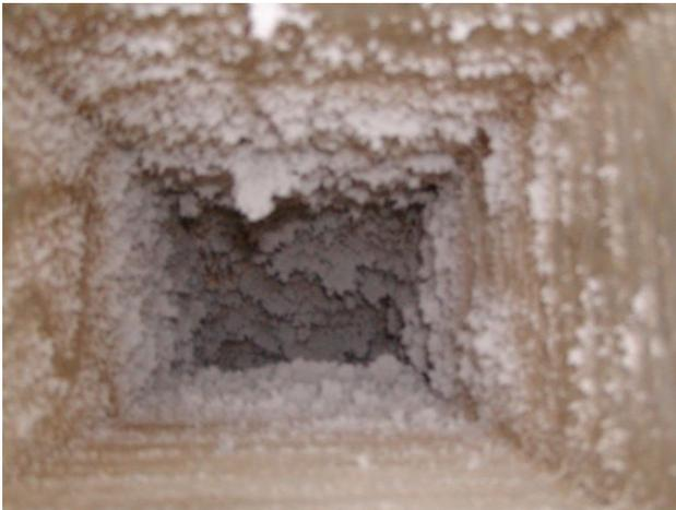
Figure 1 Particulate build-up inside ductwork.
