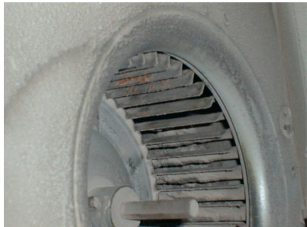
Figure 2 Particulate build-up on a blower wheel.
