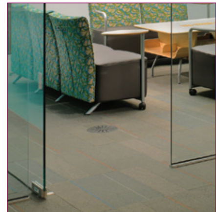
Figure 30: RFDD installed in floor
