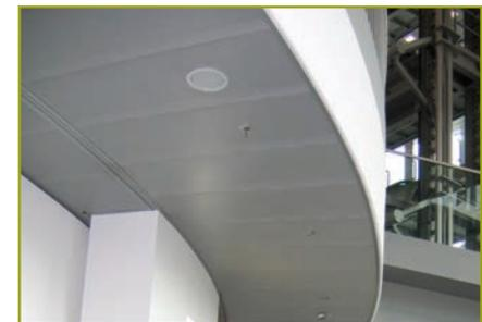
**Figure 4:** Passive beams behind a perforated ceiling
