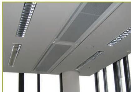
**Figure 3:** Active beams installed in an office
